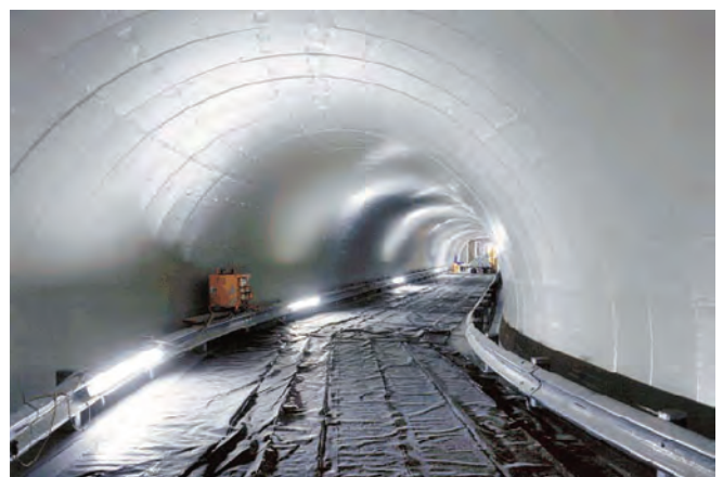
The Harrods service tunnel under construction
